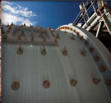
Recommissioned 1.2Mtpa Three Mile Hill Plant
